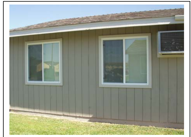
New roof, windows and exterior paint
